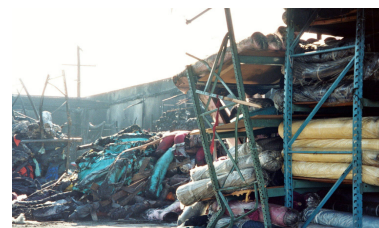
Fire sprinklers do little to protect your stock. This textile warehouse was a total loss to both building, and contents, a $3,800,000 loss.
